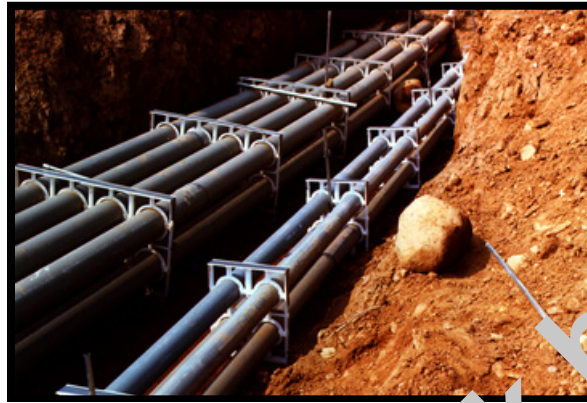
Typical Installation Using Spacers
