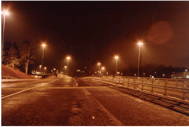
Fig. 1a - Typical roadway lighting installations. (Images courtesy of Paul Lutkevich, Parsons Brinckerhoff)
