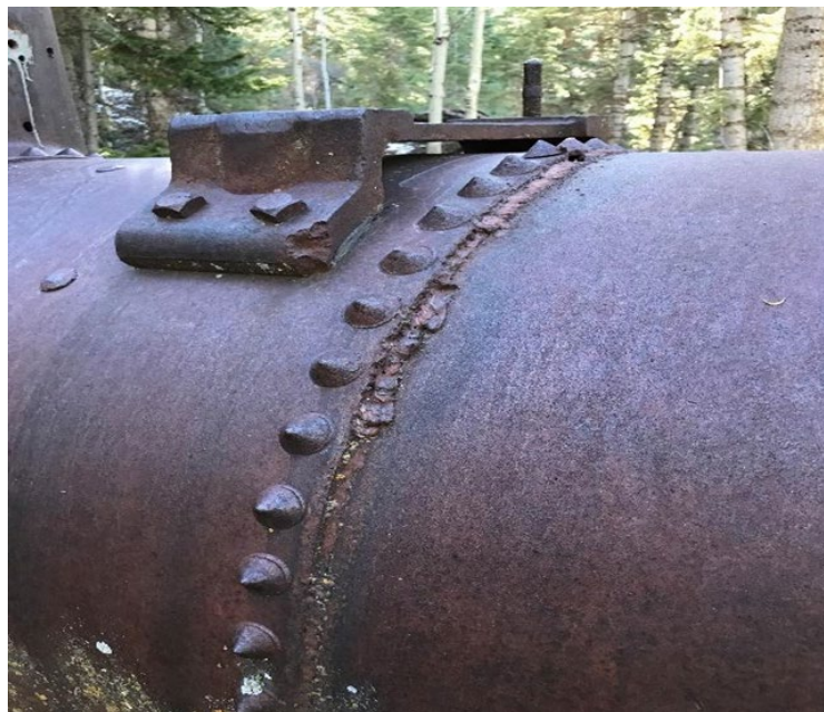
Figure 1-1: Period Repair Work on a Riveted Seam
