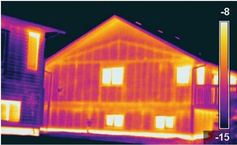
Figure 1-1. Thermal efficiency of insulated concrete form (ICF) and wood-framed houses (foreground building and background building, respectively).
