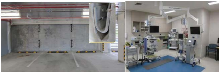
Figure 6-27. Negligible observed damage to the Southern Cross Hospital designed with a rocking-dissipative solution during the Christchurch earthquake. Source: Pampanin et al. (2011).
