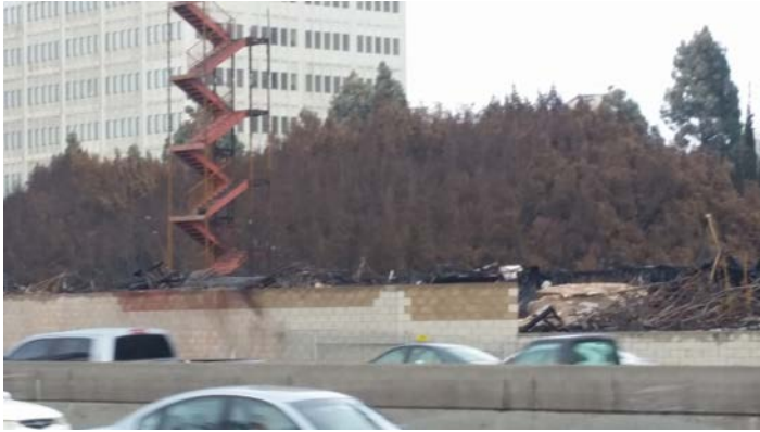
Figure 2-7. Postfire photo of the Da Vinci Complex showing only steel stairs surviving the fire.
