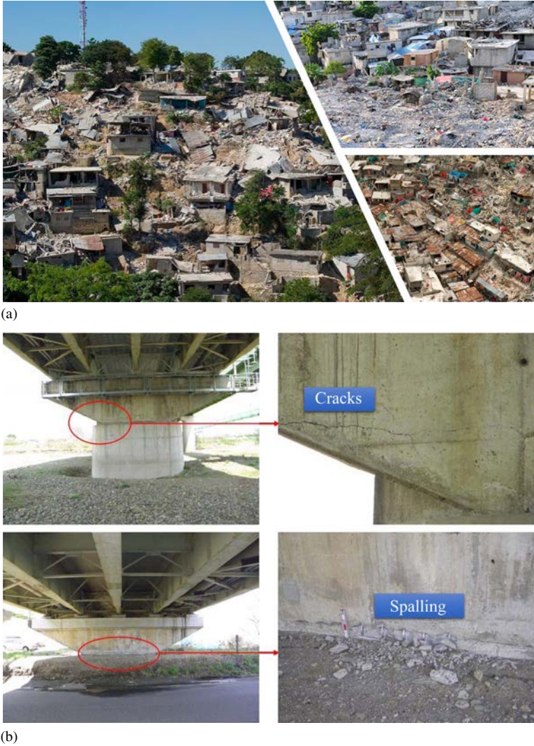
Figure 5-4. (a) Several damage scenes from the 2010 Haiti earthquake with complex terrain, and (b) a damage scene showing debris impact on a bridge pier in the aftermath of the 2011 Japan Tsunami.
