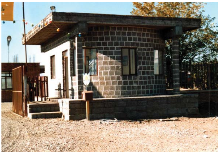
Figure 6-14. The first pure-friction base-isolated masonry building in Iran. Photo: F. M. Tehrani, LECA Plant, Saveh, Iran.
