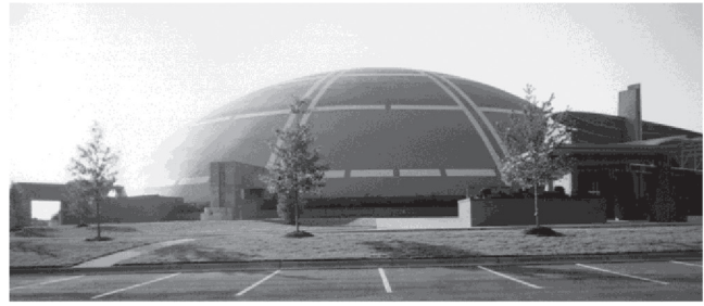
Fig. 1.1—Faith Chapel Christian Center, Birmingham, AL. 280 ft (85.4 m) diameter and 72 ft (22 m) tall, which includes a 3200-seat sanctuary, classrooms, and an administration building.
