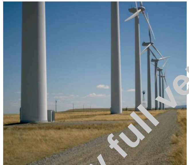
Fig. 3.1.1a—Typical row of turbines in a wind farm and their access road, Arlington, WY.
