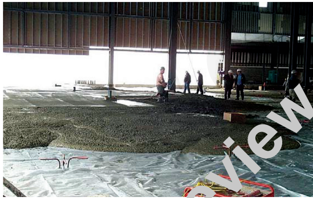
Fig. 1.1a—Installation of G-SFRC slab (pile-supported ground slab) (courtesy of Boeing Aerospace Inc.).
