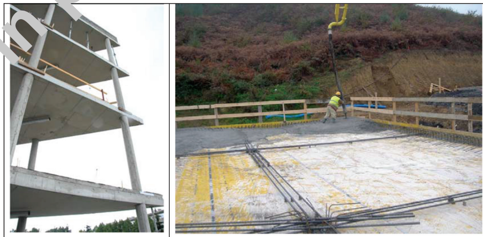
Fig. 1.1b—Construction and applications of E-SFRC slabs (courtesy of Primekss SIA).
