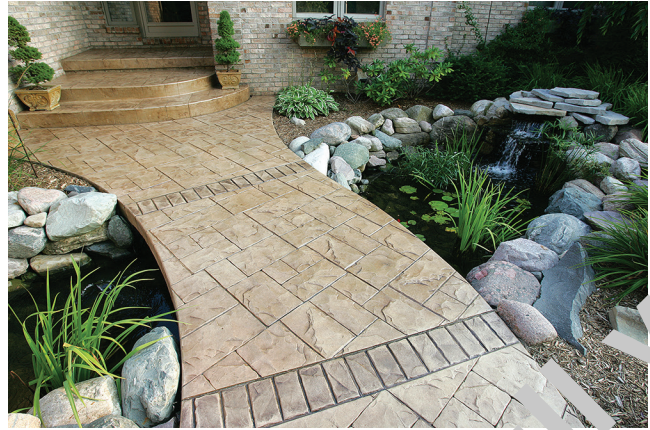
Fig. 1.1a—Stamped, colored concrete with slate and brick patterns in landscape setting (courtesy of Decorative Concrete Resources).
