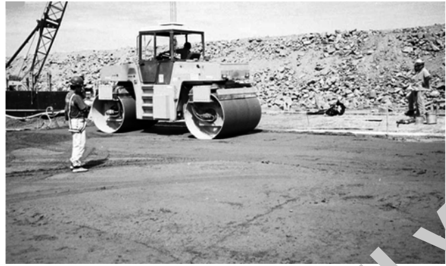
Fig. 1.1—RCC compaction with dual-drum, vibrating roller (Serra do Facão Dam, Brazil, 2008).
