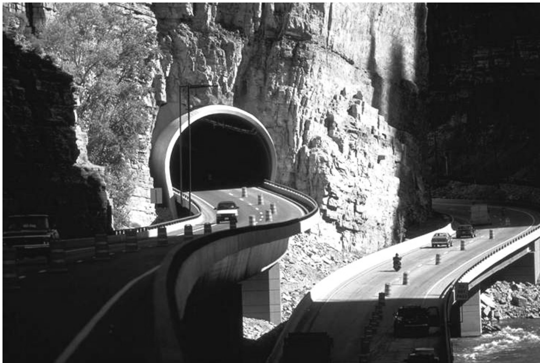
Figure 1.1-1 —Glenwood Canyon Reverse Curve Tunnel
